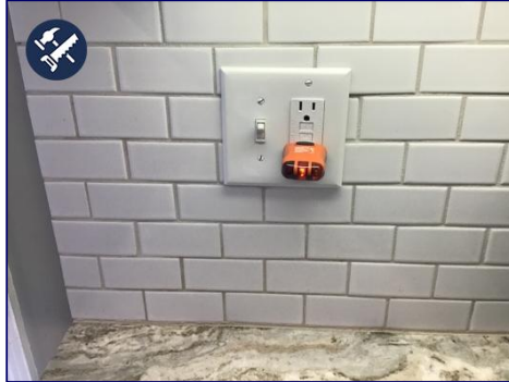
Far left of sink. Open ground, does not trip
