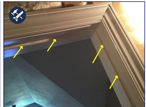
Missing insulation around attic access doorway
