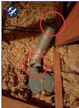
Exhaust vent missing duct from master bath
