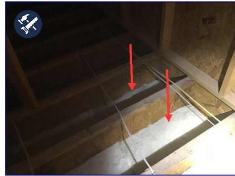
Missing insulation in main attic, left of access door.
