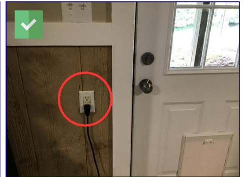
This GFCI resets the back and deck outlets.
