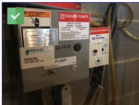
Console for pump and pump alarm for septic system.
