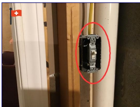
Light switch needs plate.
