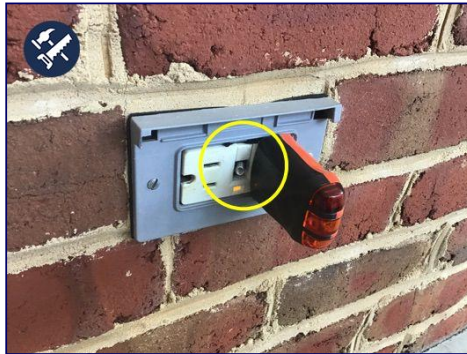
Front GFCI needs repair/replacement
