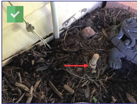
Ground rod for electrical service panel
