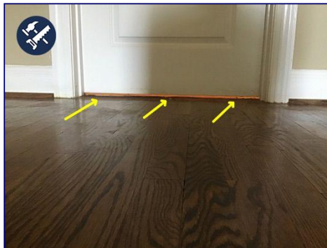
Access door missing insulation
